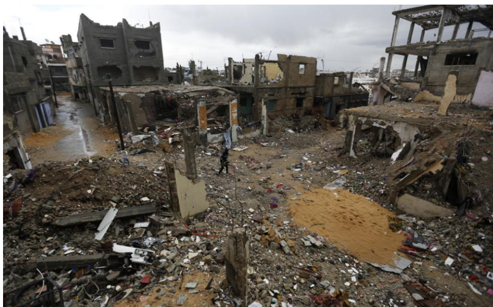
Large parts of entire neighbourhoods, such as Shujaiyeh, remain in rubble (2015).
